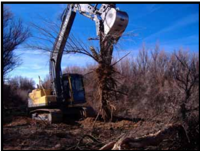
Salt cedar root being extracted mechanically along Abo Arroyo.
