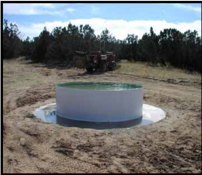
EQIP Project – Metal tank
