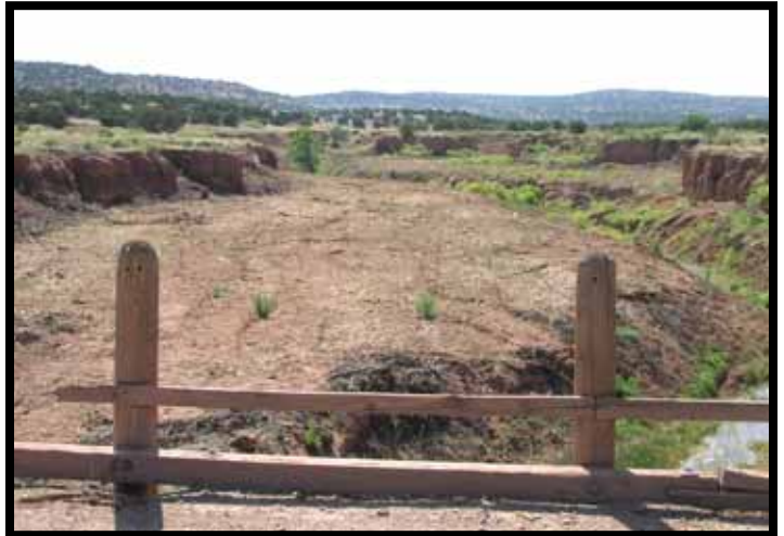
Historic Scholle Bridge After treatment.
