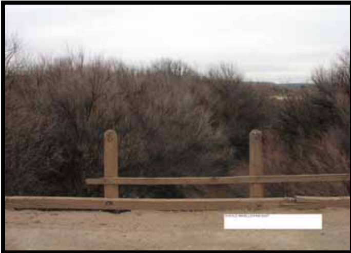
Historic Scholle Bridge before treatment.
